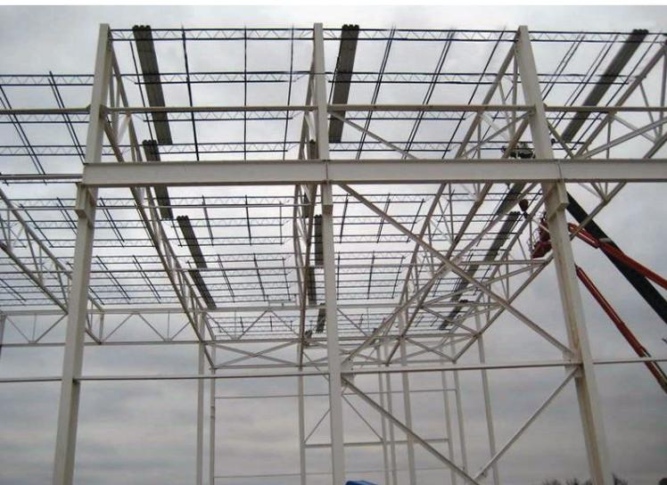
mediately braced. In hindsight, it's clear that this system “worked in the model” but wasn't conventionally constructable—a fact not noted in the design documents.
