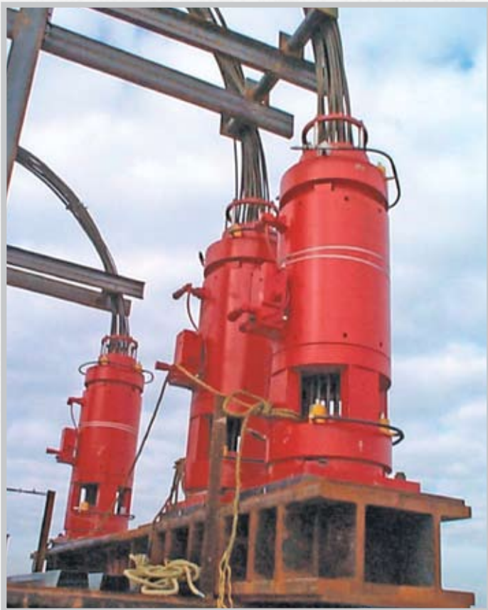
Figure 5: Strand Jack Heavy Lift Technology.
