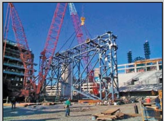
Tip up of truss assemblies
