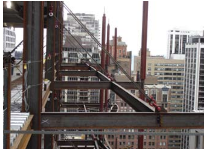
A six-story super truss, erected using a cable system, cantilevers the last bay of the patient wing from Level 14 through 22.
