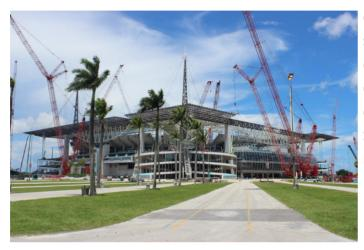
complete steel erection. To meet the project's tight schedule and overcome its unique construction challenges, Hillsdale engaged Ruby+Associates, Inc., to develop the erection procedure for the structure. As on many previous projects, Ruby turned to Tekla Structures for 3D modeling, rigging planning, clearance review and fabrication detailing.
