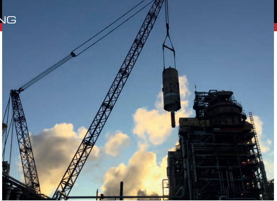
The tailing crane was a Liebherr LR-1600/2 in the SDB configuration.
