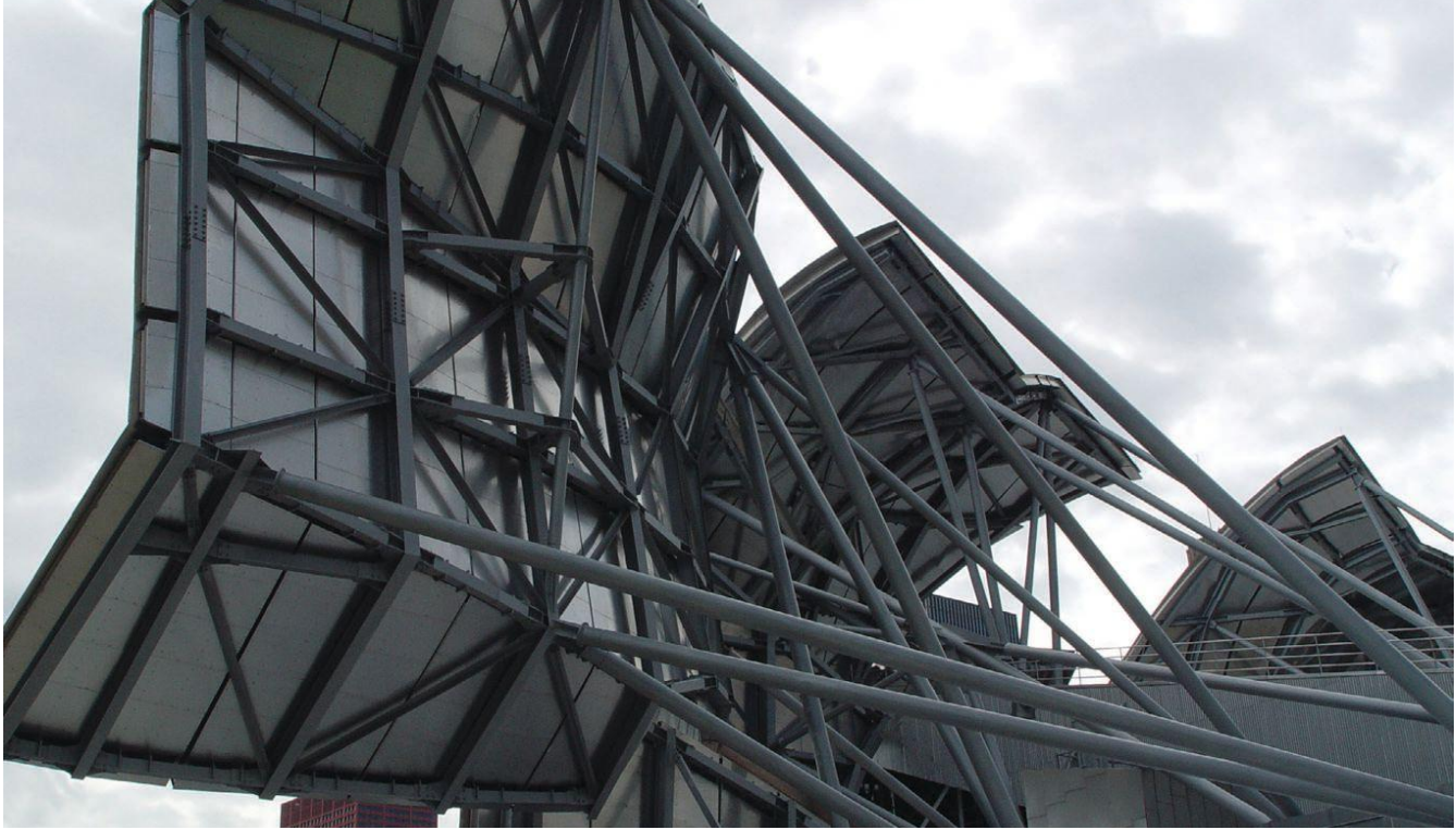
▲ Pritzker Pavilion: the structure behind the complex roof geometry.
