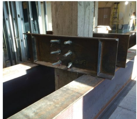
right: The system involved spreading a concrete column load using structural steel beams.
