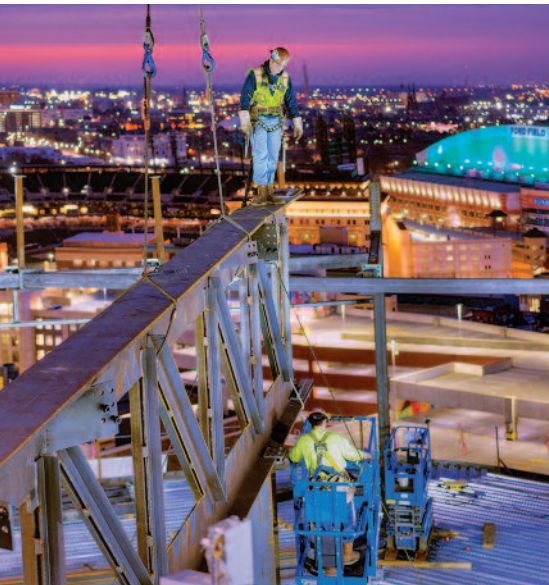
Top Left: Ironworkers stabilizing the first section of truss prior to crane release.
