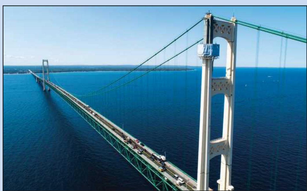
THE ONE-OF-A-KIND SCAFFOLDING used to support Seaway Painting painters on the Mackinac Bridge’s North and South towers over the past few years has been removed as the project nears completion. The platform not only allowed painters a safe and efficient base and enclosure to do their work, it was an engineering award-winner.
