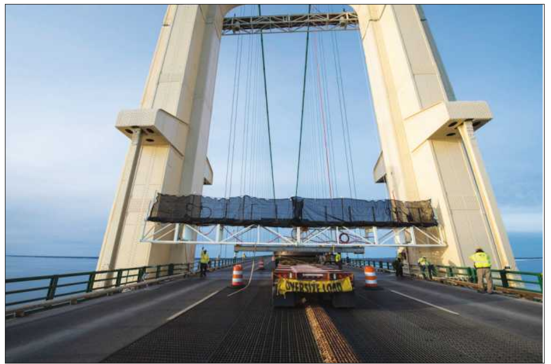
CONVENTIONAL SCAFFOLDING was used by Seaway Painting workers to paint lower parts of the 552-foot-tall Mackinac Bridge towers.
