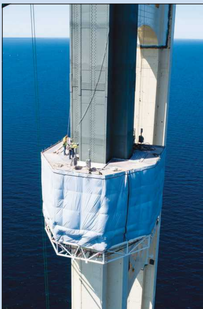
THE SCAFFOLD SYSTEM was designed to closely hug the 552-foot-tall Mackinac Bridge bridge towers, even as the towers taper as they rise. The enclosed 24-foot-tall scaffold helped allow the safe collection of old paint that was blasted off the towers. Cables suspended from new outriggers at the top of the towers allow the movement of the platform.
