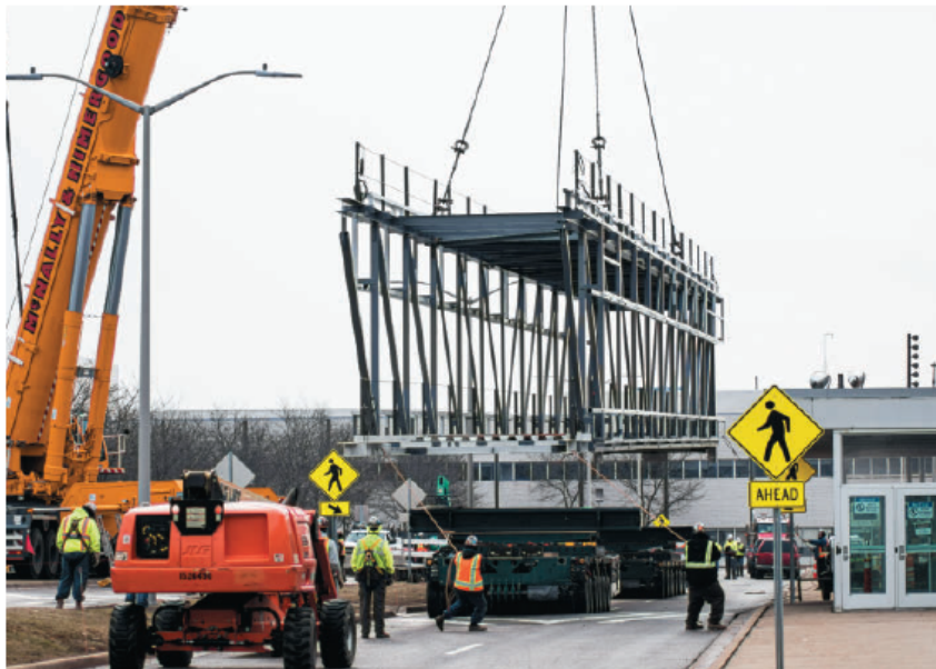
A 150-foot-long span for the Cole-Estes Pedestrian Walkway is lifted off the Goldhofer transports by a 900-ton crane, ready for installation. PHOTO COURTESY OF IDEAL CONTRACTING
